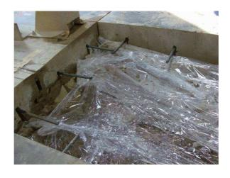
Install a HC Sinus Slide® joint in the middle of the gap opening between the concrete slabs. Level out the HC Sinus Side® joints down and across. Eventually, weld the dowels fixed in the concrete slabs to the anchorage system of the HC Sinus Slide joint or use reinforcing mesh to link dowels and joint connectors.
